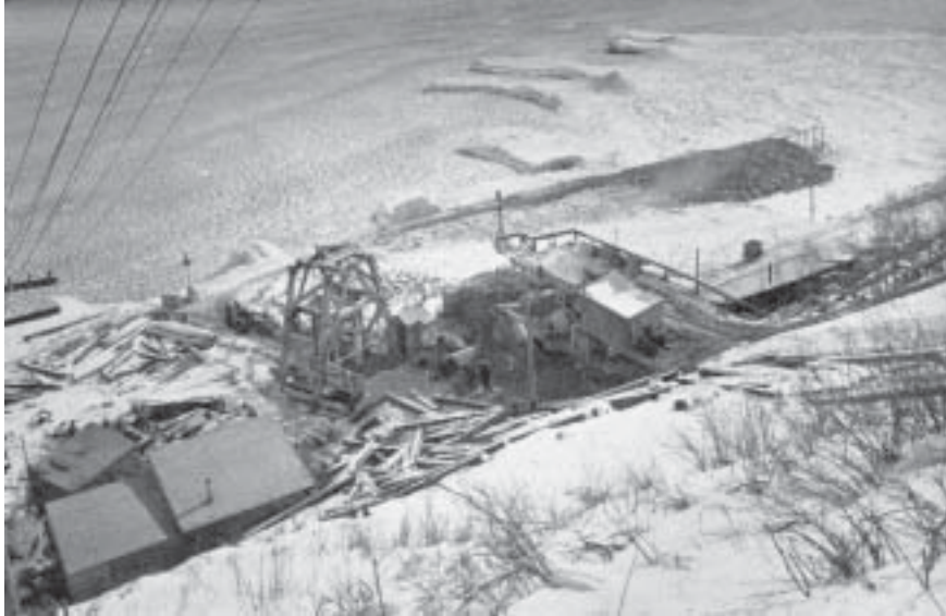
Figure 3. Shaft site and dump pile of Late Devonian rocks from which Raasch collected, the city of Milwaukee Linwood Avenue Intake Tunnel, near Lake Park, Milwaukee, Wisconsin (circa 1913; from Mesiroff, 1914).
